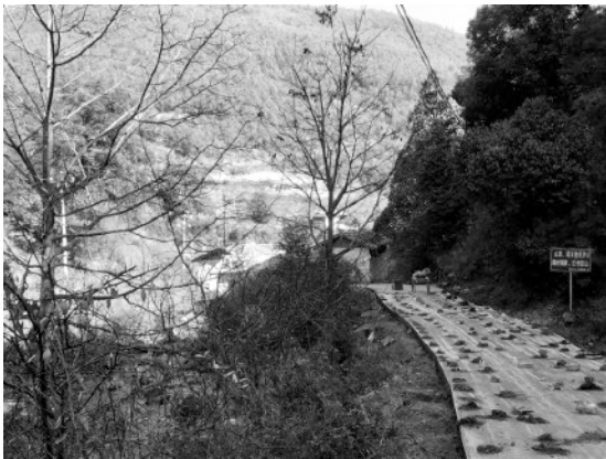
Figure 3. A secondary branch of the paved road under construction, November 2018 © The author.
